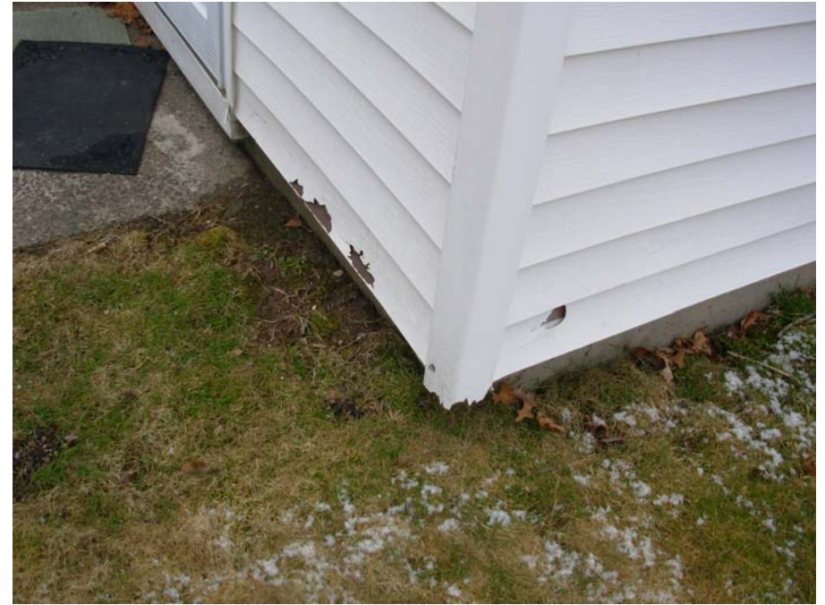
6. Most vinyl siding damage at grade levels
