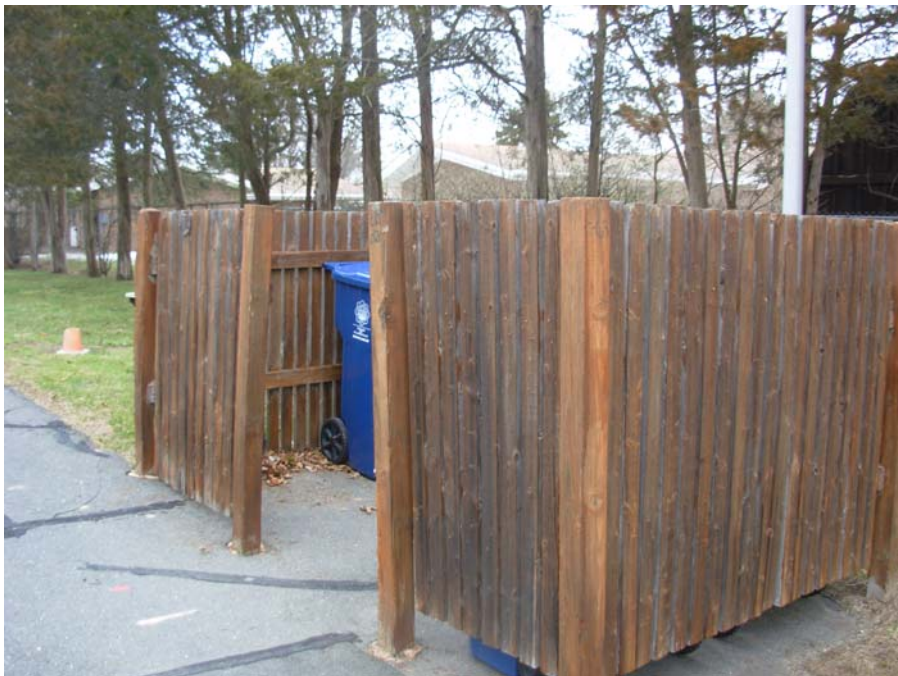
3. Some deterioration of trash can enclosure fencing
