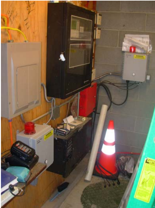
9. Fire detection and sewage ejector pump monitoring systems
