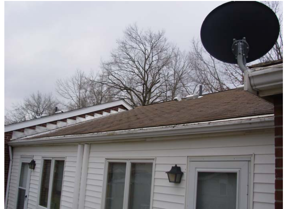
8. Lifting and curling of roofing shingles
