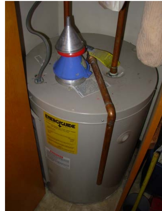
12. Electric DHW tanks serving apartments
