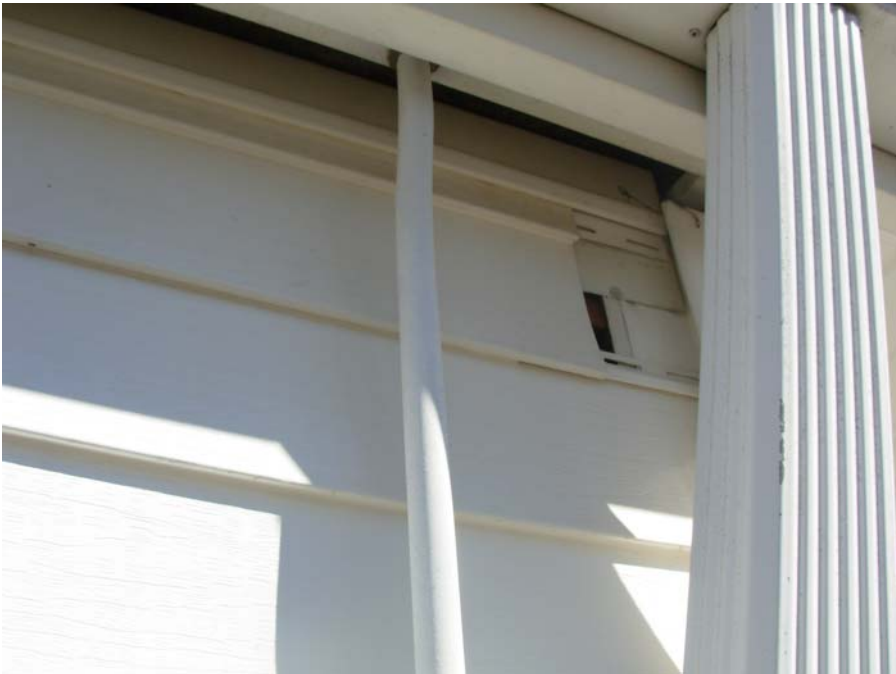
7. Spot vinyl siding damage at soffit areas
